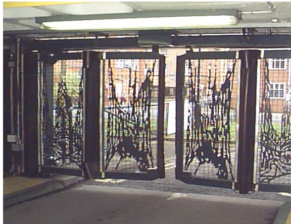
Figure 2: Gates to the car park
