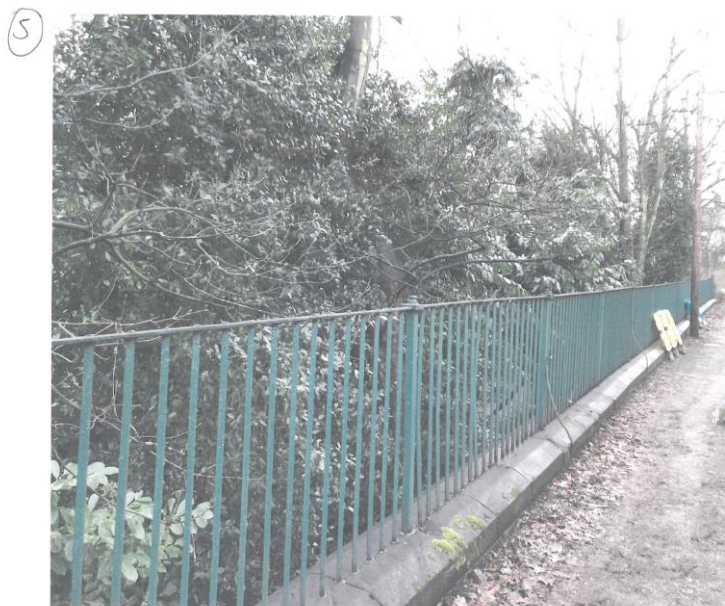
Figure 3: One of the participant's photographs which depicts the lack of visibility into the site
